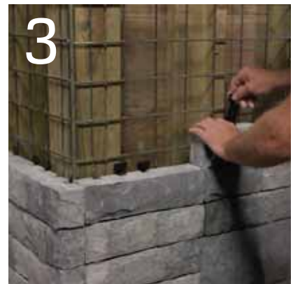
3 Attach Tandem Veneer with Connector
